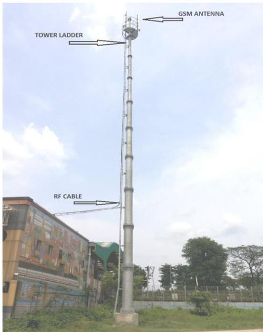
Site configuration of BTS is 2 TRX per site for most of the stations except for Metro Bhawan where BSC has been taken as 3 TRX per site. GSM-R system covered all the 15 tunnel stations & 9 via duct/surface stations and Metro Bhawan. Two Core Dispatcher are installed, one in Metro Bhawan for Traction Loco Control and another one in Noapara Car shed for PPO. Cab Radio is installed in Rake for the Cab Drivers.
