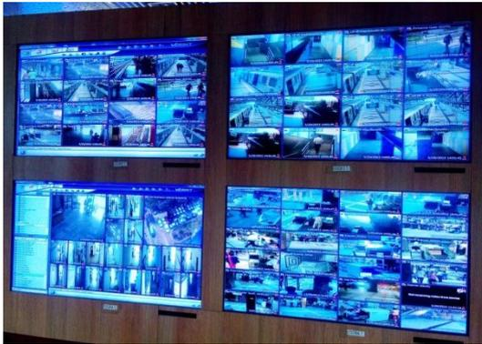
Apart from monitoring arrangement provided to the Station Masters to view feed from cameras fitted in their respective station, a centralized monitoring arrangement has been commissioned in Metro Bhavan where feed from the entire 662 cameras can be monitored and recorded round the clock for improved security surveillance and investigation on the Metro system. Pan,
