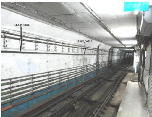
Leaky cable laid in tunnel section is used to provide network coverage in tunnels. For coverage in via-duct portion, antenna has been fixed on Tower. All equipments have been installed and are working. GSM-R Construction work started in February 2013 and completed in 15<sup>th</sup> August 2014.
